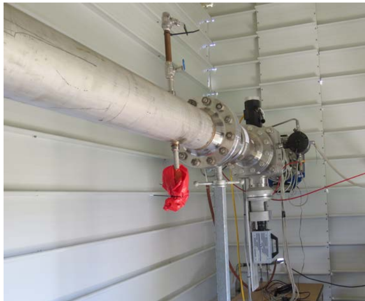
Figure 4. Closed up view on the instrumentation installed at the test section
